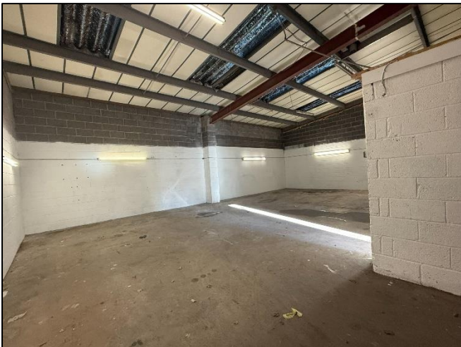
Warehouse (prior to refurbishment)
