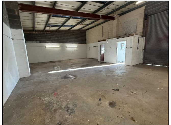
Warehouse (prior to refurbishment)
