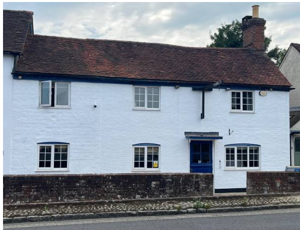
No 87 – Ground & 1 st Floor Office
