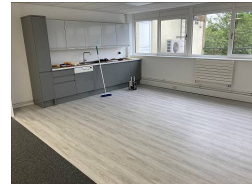
Newly fitted kitchen
